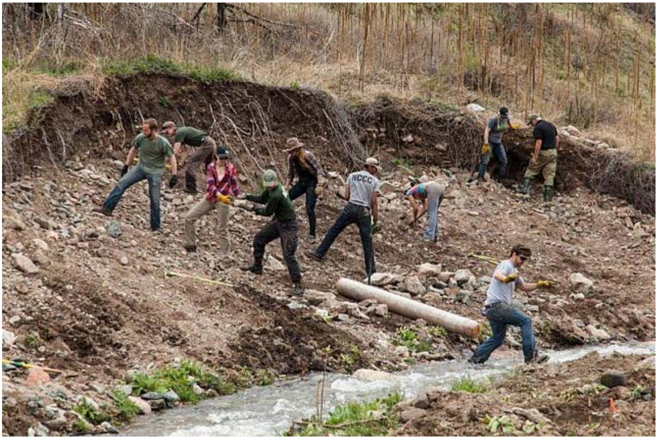
WRV volunteers prepping an unstable stream bank
